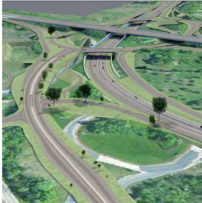
Figure 16: Image of the Raith Interchange project in Scotland. (Scottish Futures Trust)
